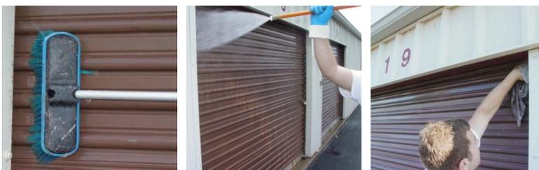
**Prior to applying any top coat re-inspect. If dust, chalk, or dirt remains, repeat the clean/etch process!**
